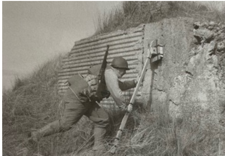
Figure 7 Attaching pole charge to bunker 696
