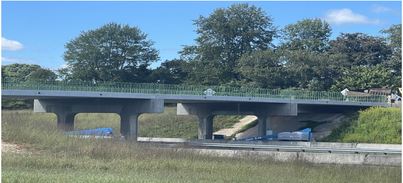
Figure 1. Causby Road Bridge construction project, September 2023. Photo courtesy of John Terry
