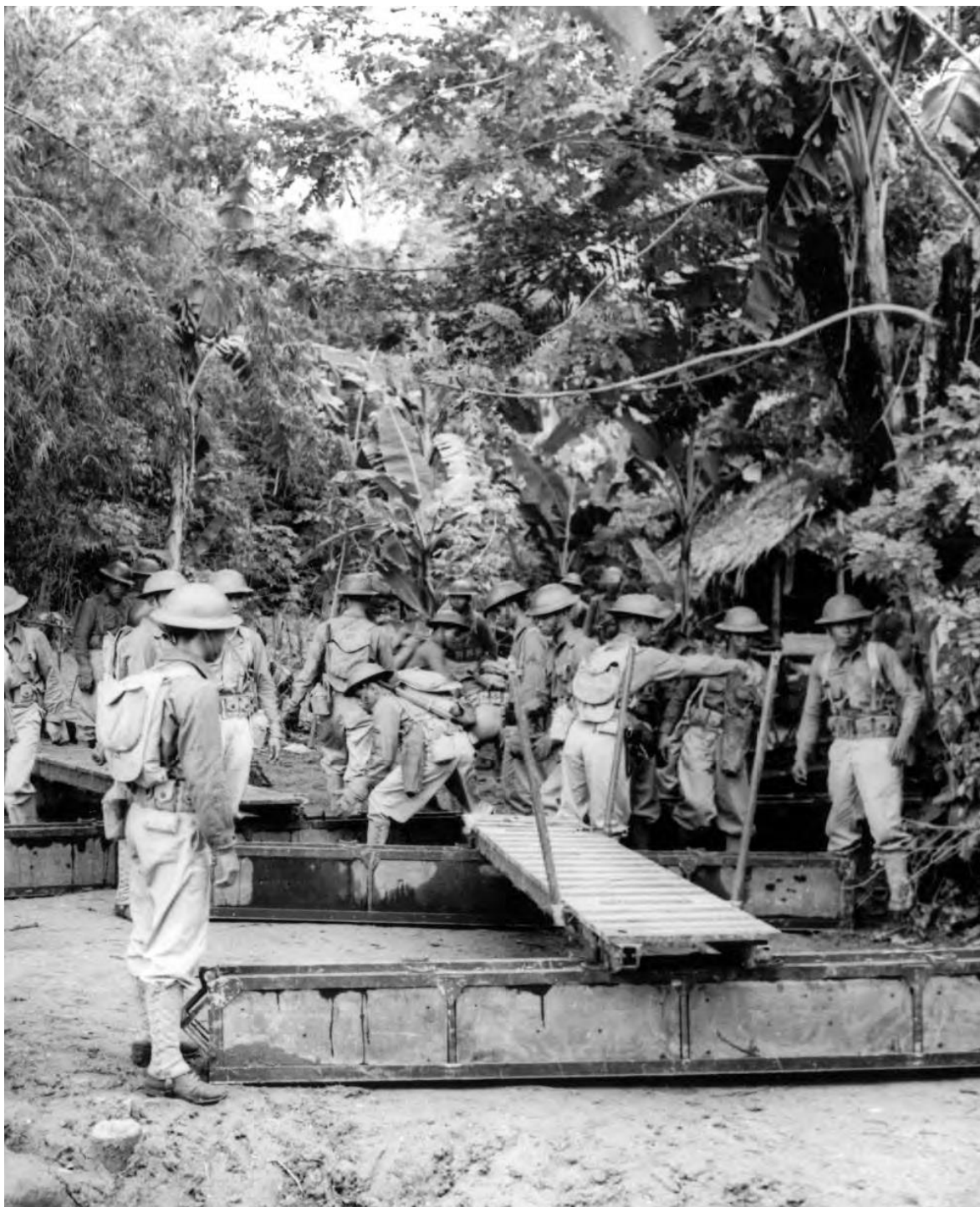
Figure 1: Engineer soldiers emplacing ponton bridge sections in position during a river-crossing maneuver in the Philippines, 1941. from: U.S. Army in War World War II: Pictorial Record, The War Against Japan , 2 nd ed. (Washington, D.C.: The U.S. Army Center of Military History, United States Army, 2001), 28.
