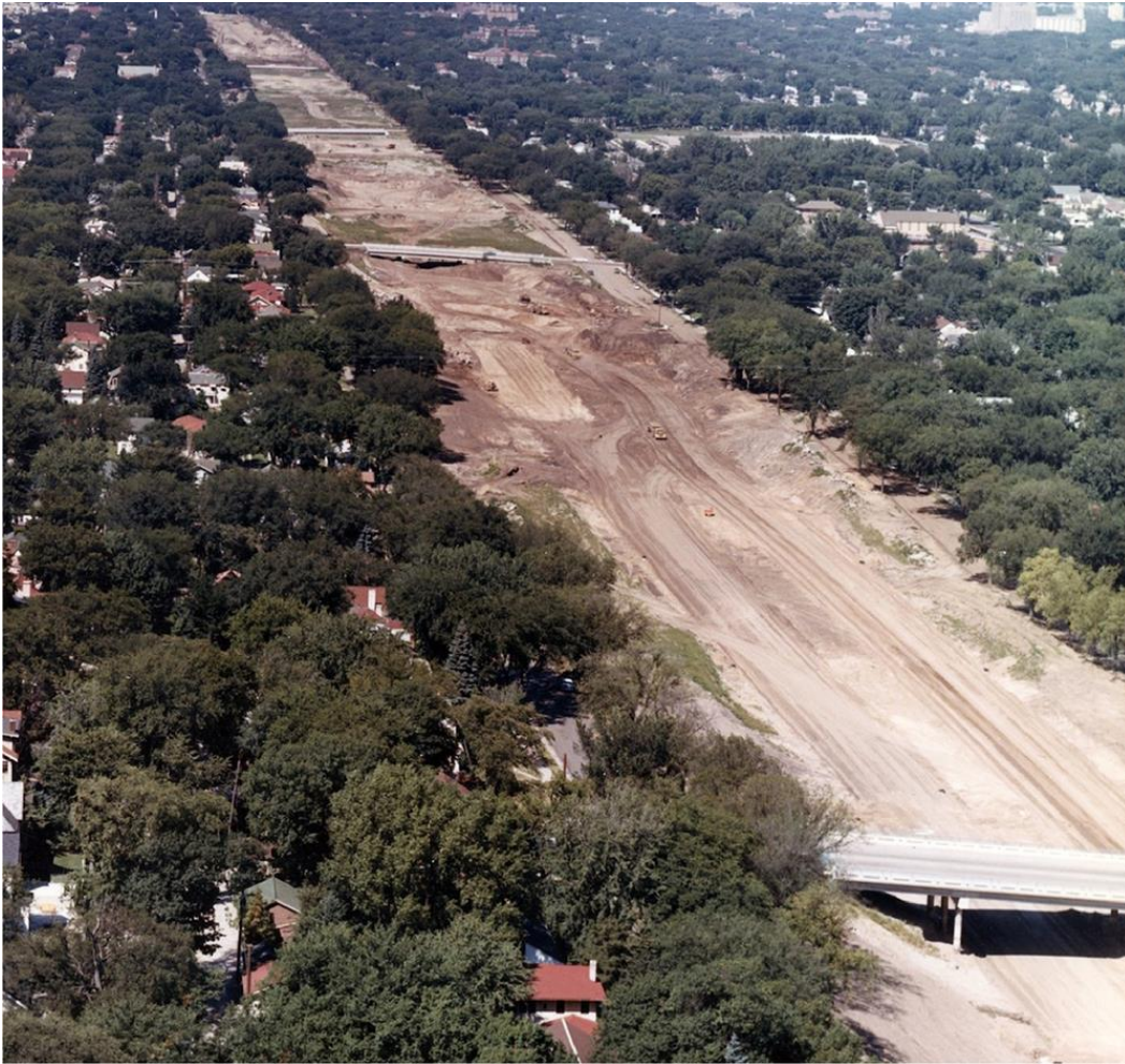
Figure 4.4 The trench excavated for 35W in South Minneapolis.
