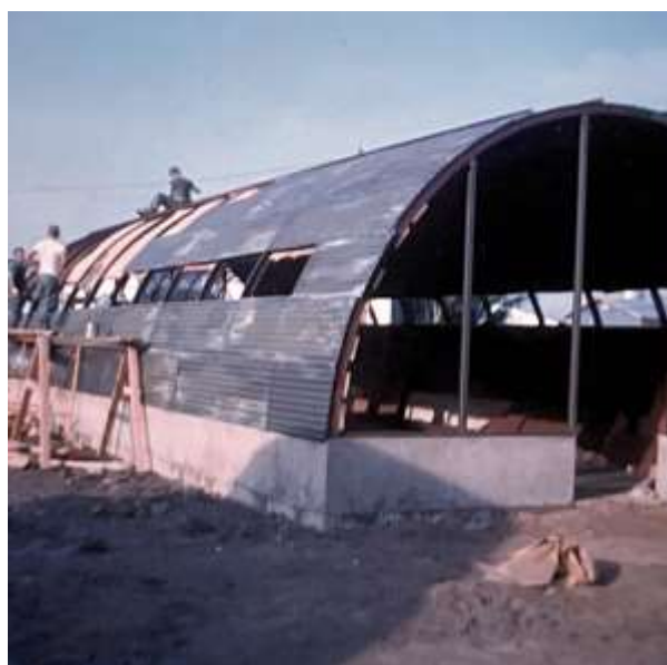
Figure 6 More Construction of WAC Quonset huts, Tan Son Nhut Air Base, FIC.2011.317, Box 634D, Betty Benson, Mag No 4, Nov 1966- Dec 1967, Photos 1-7, Photo by Betty Benson, U.S. Army Women's Museum, Fort Gregg-Adams.
