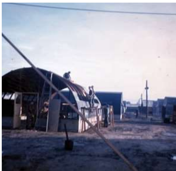
Figure 7 Construction of a Quonset hut, Tan Son Nhut Air Base, FIC.2011.317, Box 634D, Betty Benson, Mag No 4, Nov 1966- Dec 1967, Photos 1-7, Photo by Betty Benson, U.S. Army Women's Museum, Fort Gregg-Adams.
