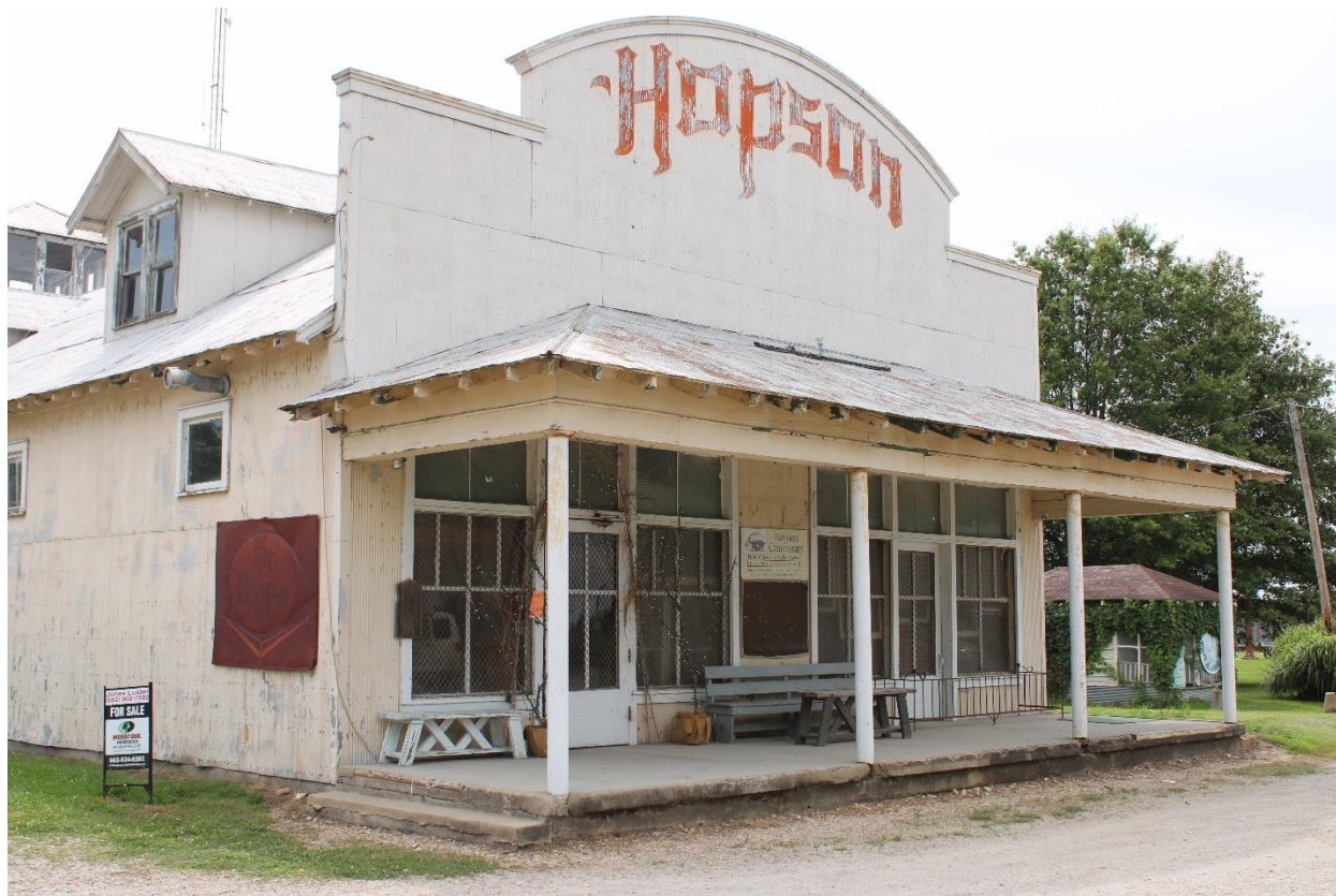
Figure 1. Hopson Commissary . Photograph by author, June 16, 2023.
