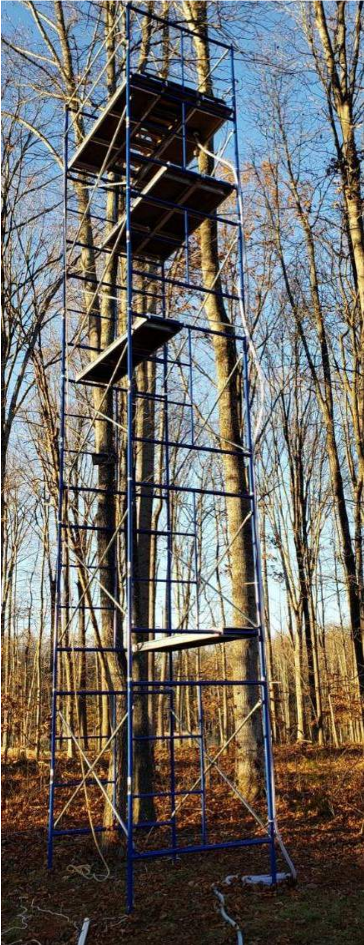
FIGURE 3.4: Scaffolding with UDCN Bladder Tank and Connections
