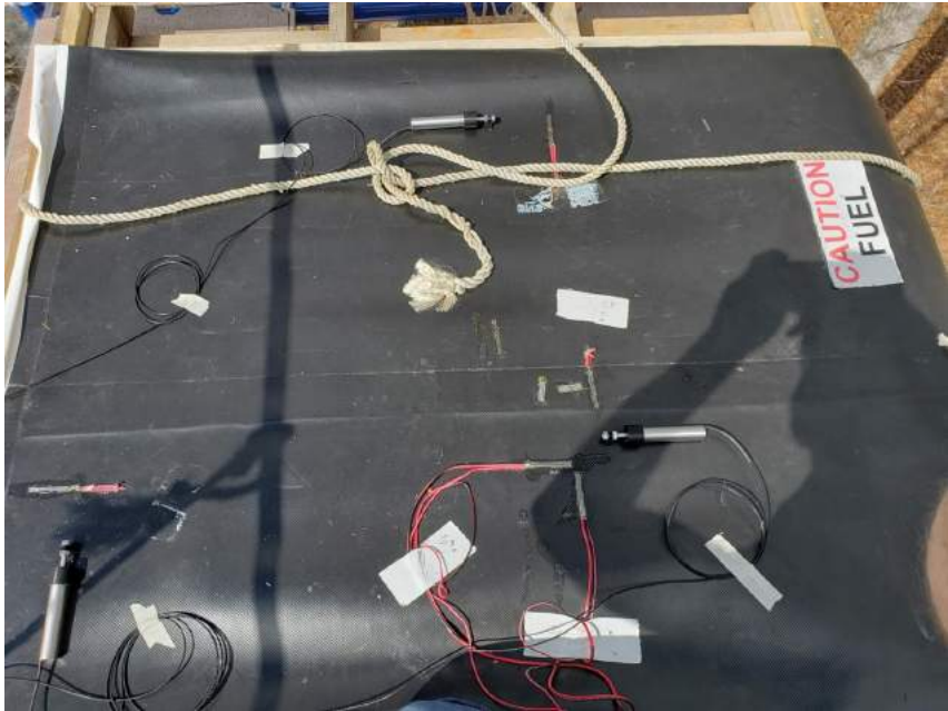
FIGURE 3.7: UDCN Membrane Tank with Sensors and Security Rope
