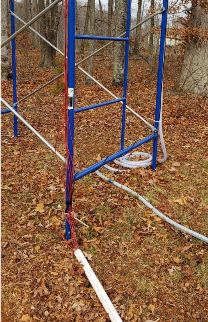
FIGURE 3.5: Sensor Wiring, PVC Conduit and Hydraulic Tubing
