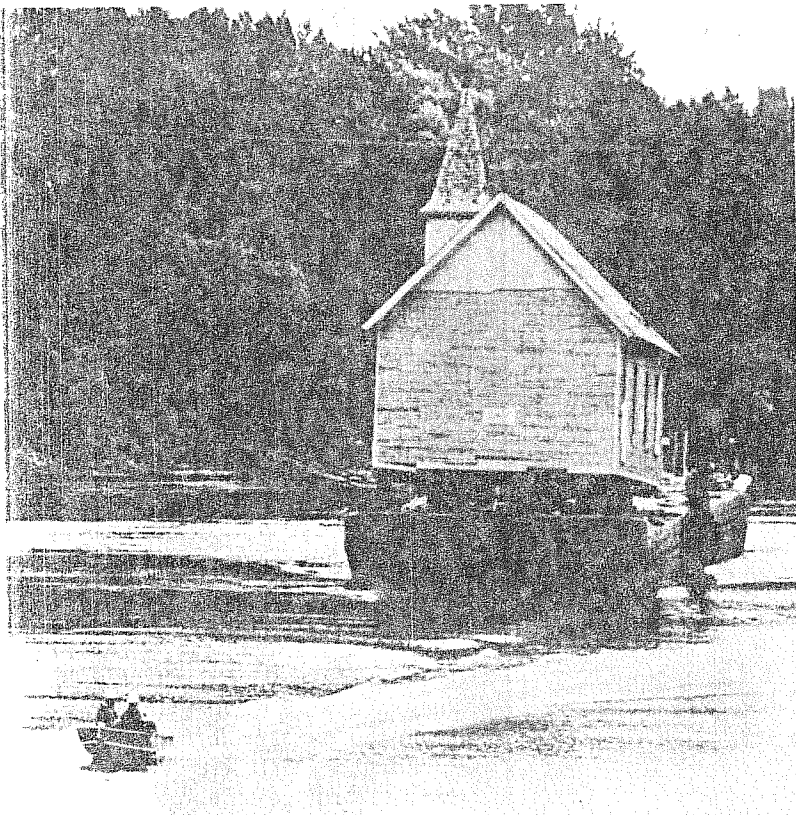
A 106-year-old Methodist Church is moved via motor boat to a Scott County historical site near Shakopee, Minn.
