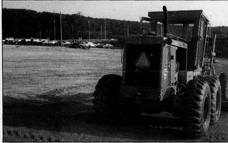
BULLDOZER — Paving for the pit continues.
